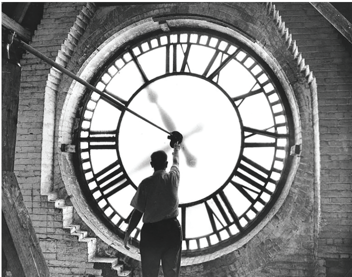
fig. 1 Fort Street Union Depot Clock, 151 W Fort St, Detroit, MI 48226, opened in 1893, demolished in 1974 © Detroit Free Press Archives
