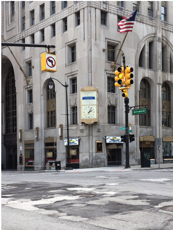
fig. 2 - Penobscot Building, 645 Griswold St, Detroit, MI 48226 © Leonie Hagen
